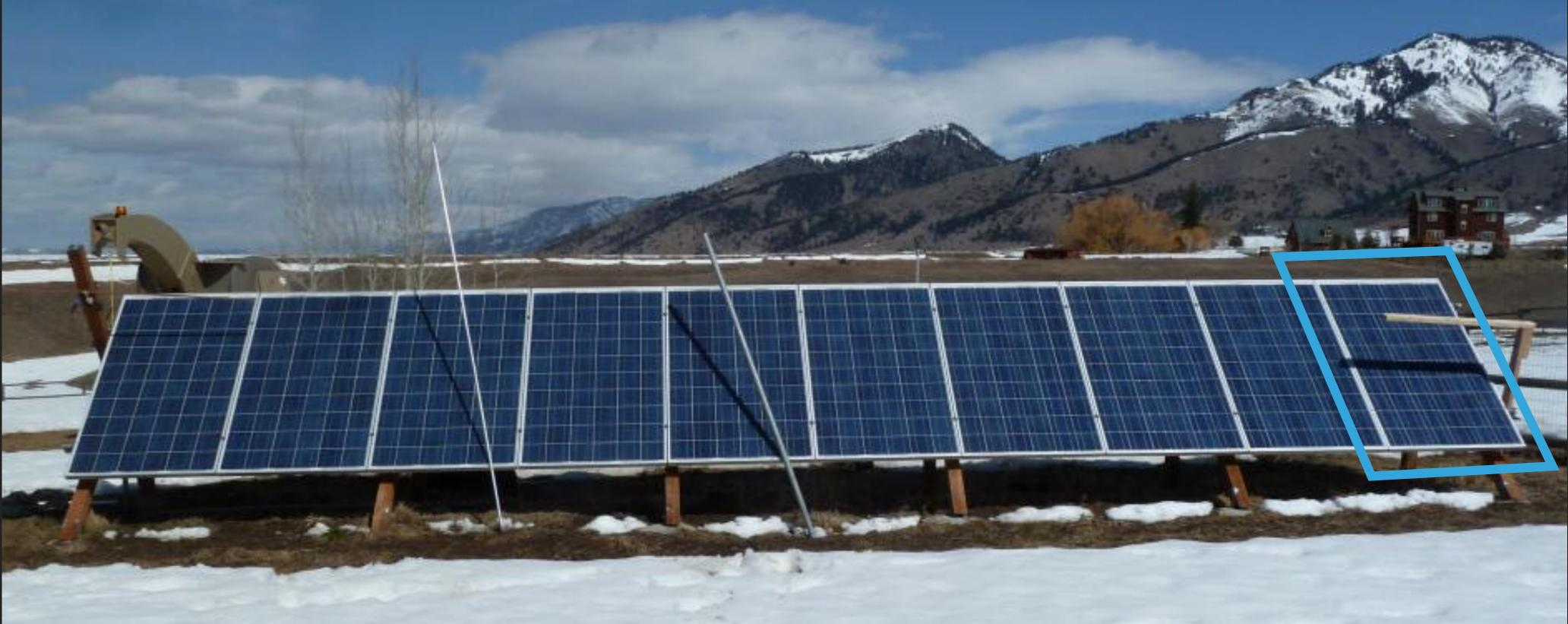
Solar panels typically consist of several cells in series. Like kinking a hose, shading one cell reduces the effectiveness of the entire series string.
