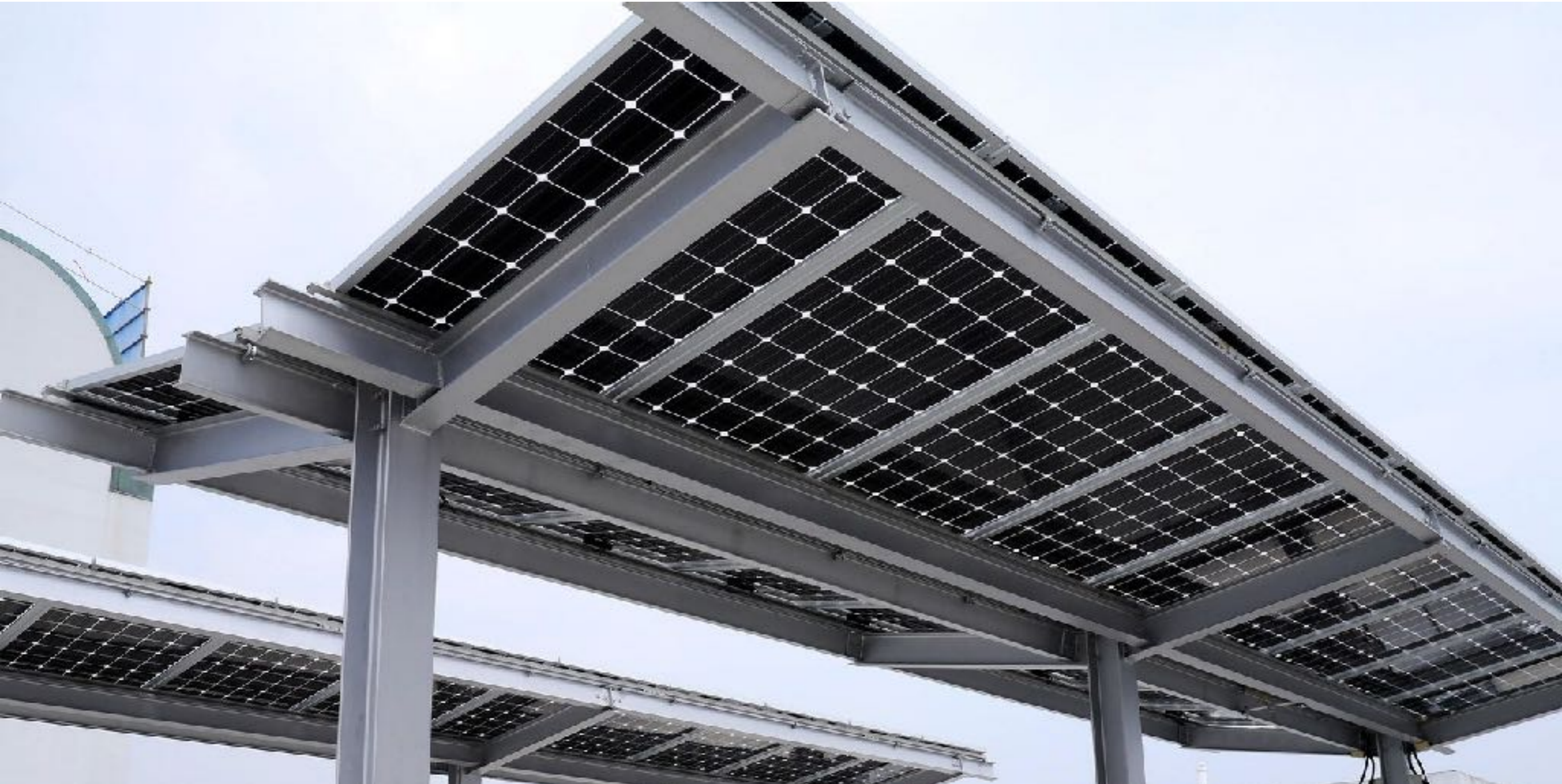
Figure 1 Unlike conventional p-type silicon PV cells, SolarWorld's PERC cells have rear passivation layers of amorphous silicon. These rear passivation layers not only improve light-trapping properties — by reflecting light at the cell boundary back into the cell — but also make the PERC cells inherently capable of bifaciality. Moving from a fully metallized rear electrode (on left) to one that is selectively metallized (on right) allows light to reach the back side of the bifacial cell.
