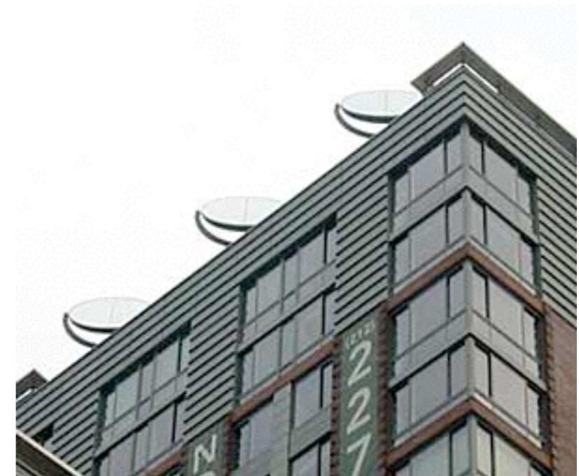
Solar lighting: Teardrop park heliostats Carpenter Norris Consulting Inc.
